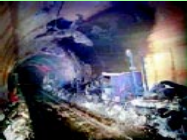
Mont Blanc Tunnel, France - 1999
