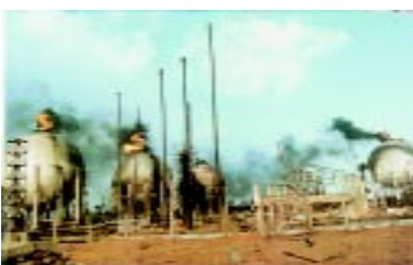
Refinery Fire, India - 1997
